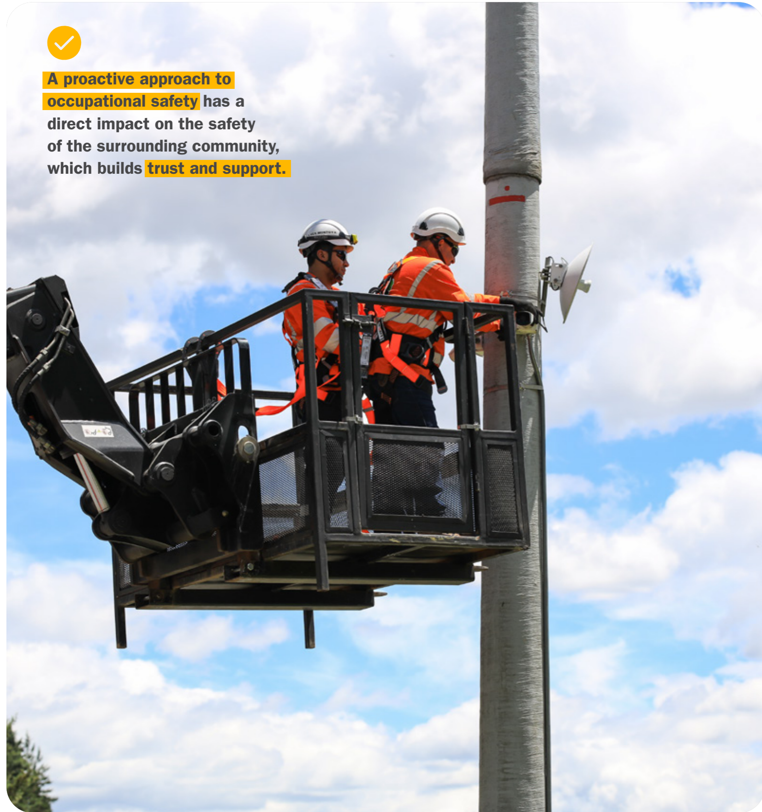
Maintenance work on road infrastructure.
